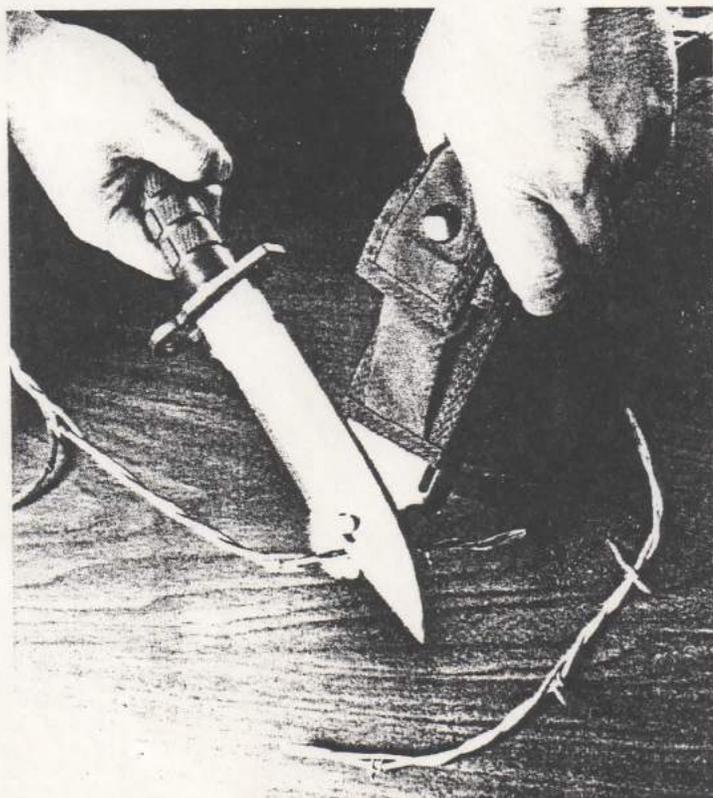
By hooking the blade around a small knob on the scabbard, the bayonet also can be used as a barbed wire cutter.
